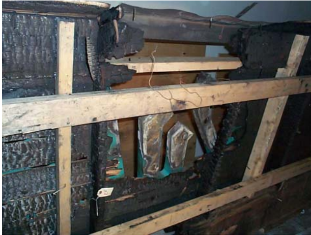
Rear of wall
